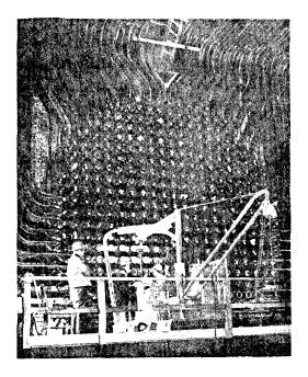
Figure 13 Installing Closure Plugs
