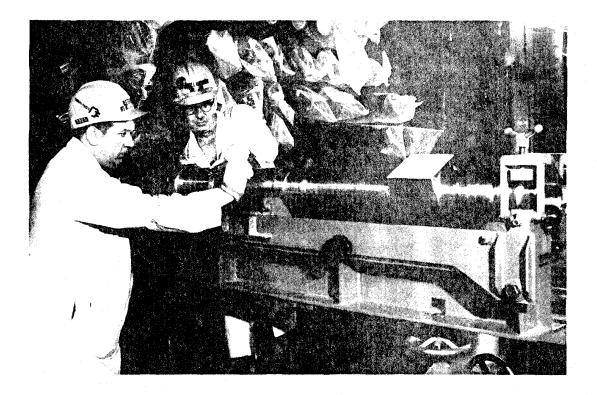
Figure 11 Installing Calandria Tube End Fittings
