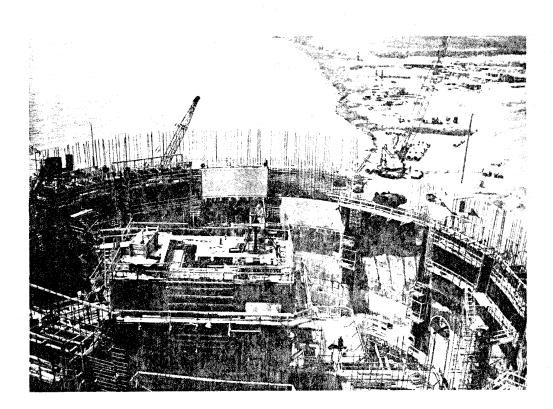
Figure 5 Reactor Building Perimeter Wall Forms and Calandria Vault Construction
