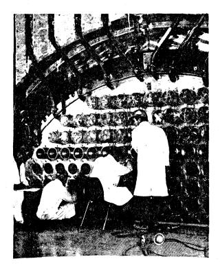
Figure 10 Calandria Tube Sheets Showing Bellows Seal
