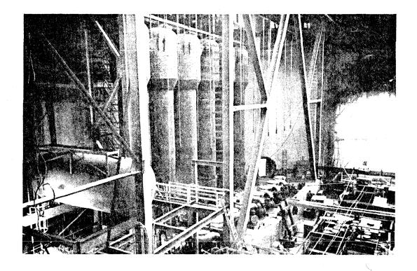
Figure 14 Boilers and Primary Pump Bowls
