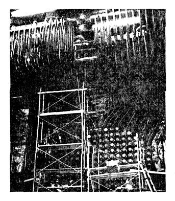
Figure 12 Feeder Tube Installation
