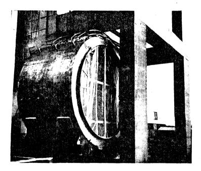
Figure 9 Calandria Being Moved into the Reactor Building
