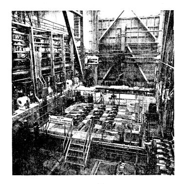
Figure 15 Reactivity Mechanism Louvers to Pressure Relief Duct in Background
